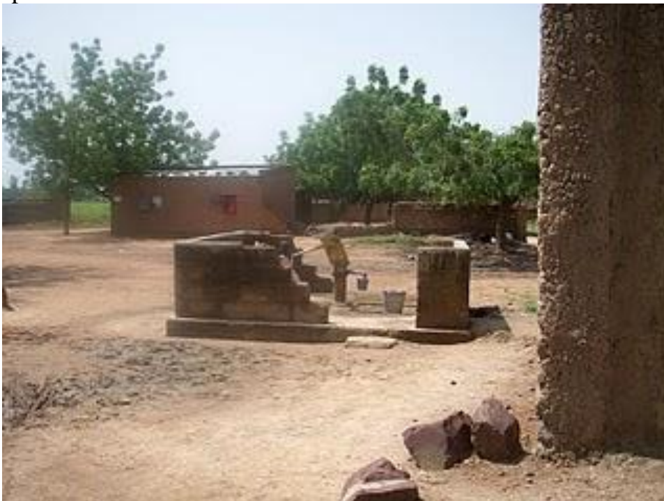
The water pump
